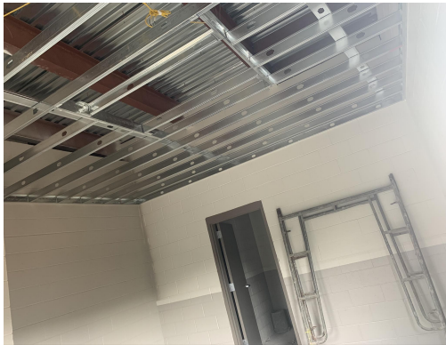
CSK- Concession Interior Metal Studs Install
